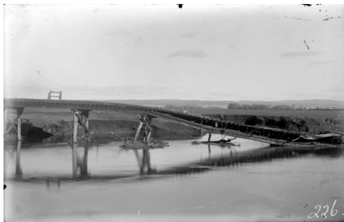
The railway bridge over the Molonglo River, showing destruction of the trestles by floods on 26-27 July 1922 (Mildenhall collection/ National Archives of Australia)
