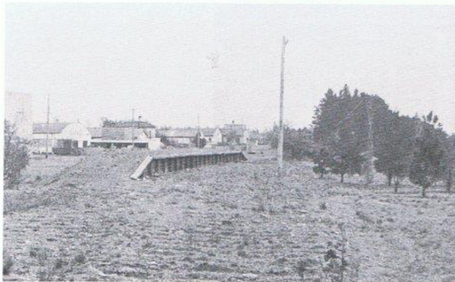
Civic Centre platform of the 1921-22 construction railway, after the rails had been lifted. Construction was of timber facings backfilled with soil. Photo: B.T. Macdonald
